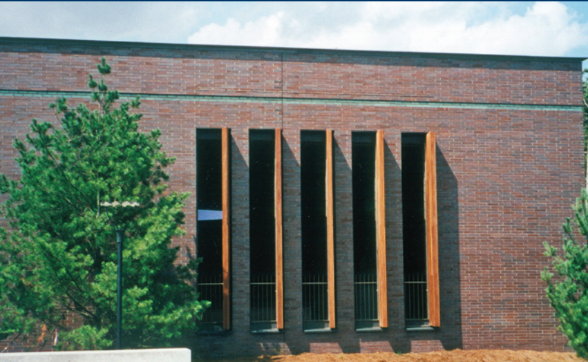
Swing Design Hydraulic Louvers in the Cranbrook Natatorium, Cranbrook Educational Community in Bloomfield Hills, MI. EPD louvers are all custom designed to match the building design.
