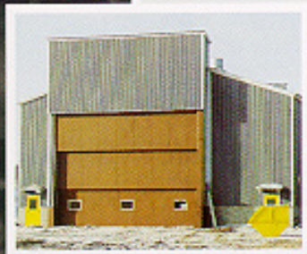
240-TON MINING HAULAGE TRUCK FACILITY OPERATES IN ALL CONDITIONS
