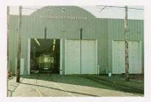
The Waterfront Streetcar Barn in Seattle, Washington, has four 14' x 16' Four Fold Doors manufactured by Electric Power Door. The heavygauge steel construction holds up well against rust in the facility near Puget Sound.
