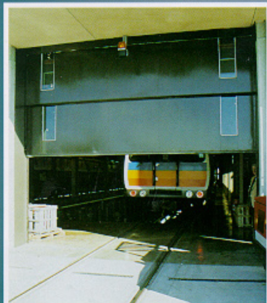
TRANSIT MAINTENANCE FACILITY
