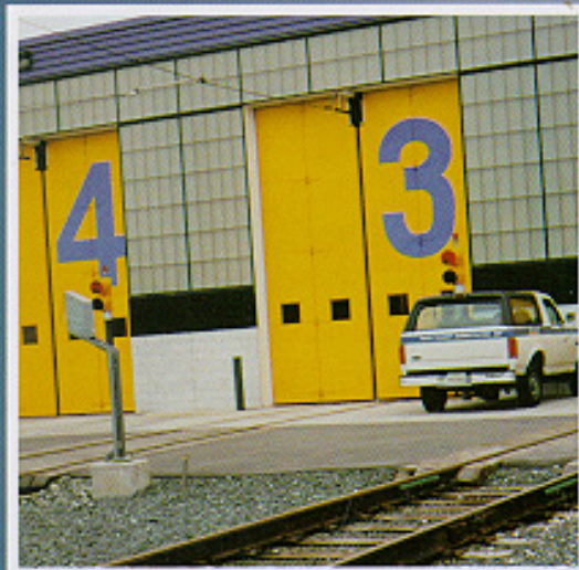
LIGHT RAIL MAINTENANCE SHOP
