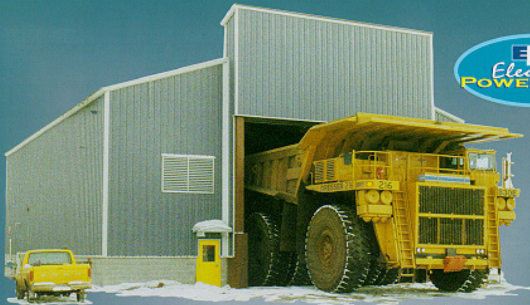
EXTERIOR MOUNTED TRUCK SHOP DOOR
