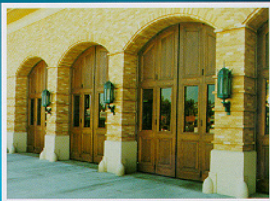
OAK CLAD FOLDING DOORS - FIRE STATION
