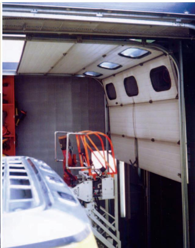
are required to install large vision panels in apparatus doors, a process that is easy in overhead sectional doors but not in rolling steel doors.
