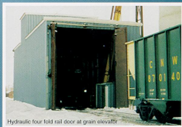
Hydraulic four fold rail door at grain elevator
