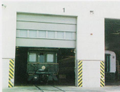
Rail repair facility for New Jersey Public Transit, Kearney, NJ. Twenty-four four-leaf Vertical Lift Doors are on the facility. The opening size on all doors is 17' x 22'.
